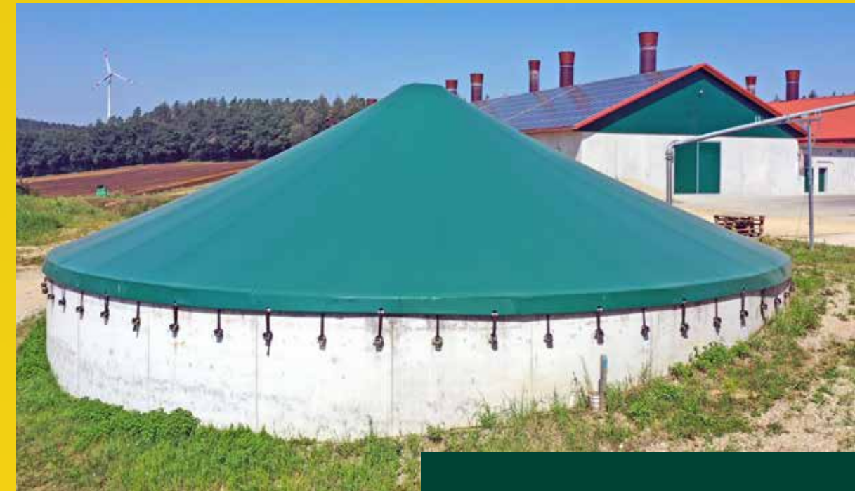
Membrane roof with central support
