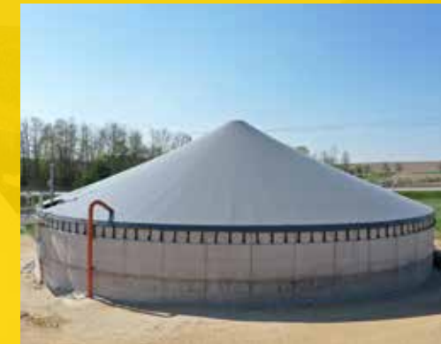
Membrane roof with central support
