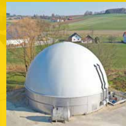
50 %-DMGS on steel container
