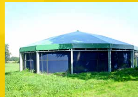
Free standing domed roof on supports
