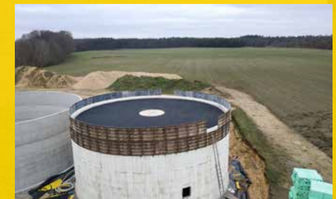
Concrete reservoir with reinforced concrete ceiling
