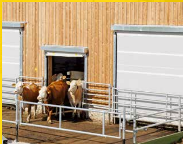
Doors at a dairy cattle barn
