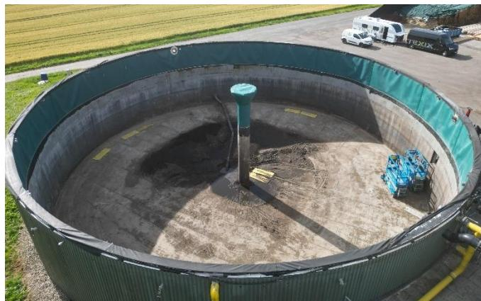
Biogas tank with SaniTarp® concrete refurbishment on the upper third of the tank wall and central support (gas space)
