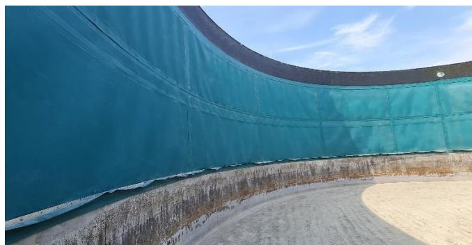
SaniTarp® concrete protection on the tank interior wall including crown protection, stainless steel clamping, and welded seam installation
