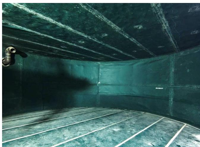
Floor, ceiling, and wall refurbishment inside biogas tank with SaniTarp® – complete internal concrete protection
